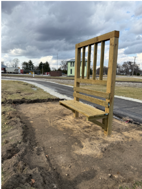
Kiosk core structure on March 6, 2026
