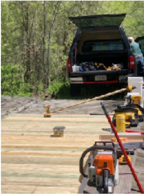
Facing east —bridge rehabilitation is underway. The left image depicts materials with tools and the placement of new perpendicular timbers nearing completion on the north half of the bridge . The right image depicts the primary crossing's diagonal timbers and Bruce and Paul working on the north half. (Image by Kathy Lucas)
