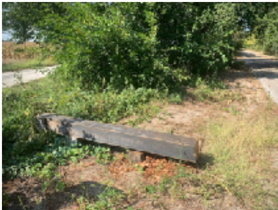
Horizontal at Starke County Road 700 South following work by Paul Byer
