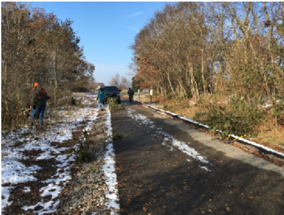
Joint workday in progress facing west (November 16, 2019) Image by Erica Luchik.
